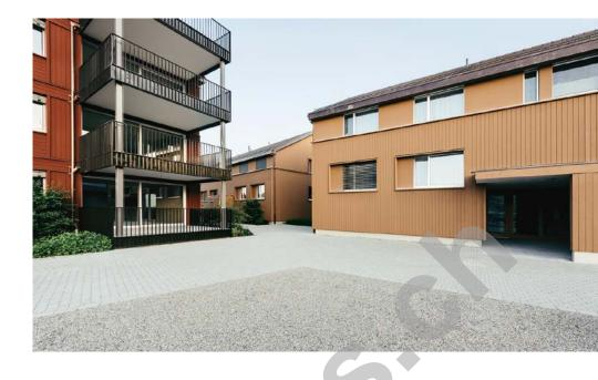
had to be guaranteed, which generated considerable outlay. This led to the facade ultimately being given four coatings: each board was waterproofed twice by the manufacturer in the factory and then given two more coatings on site.
